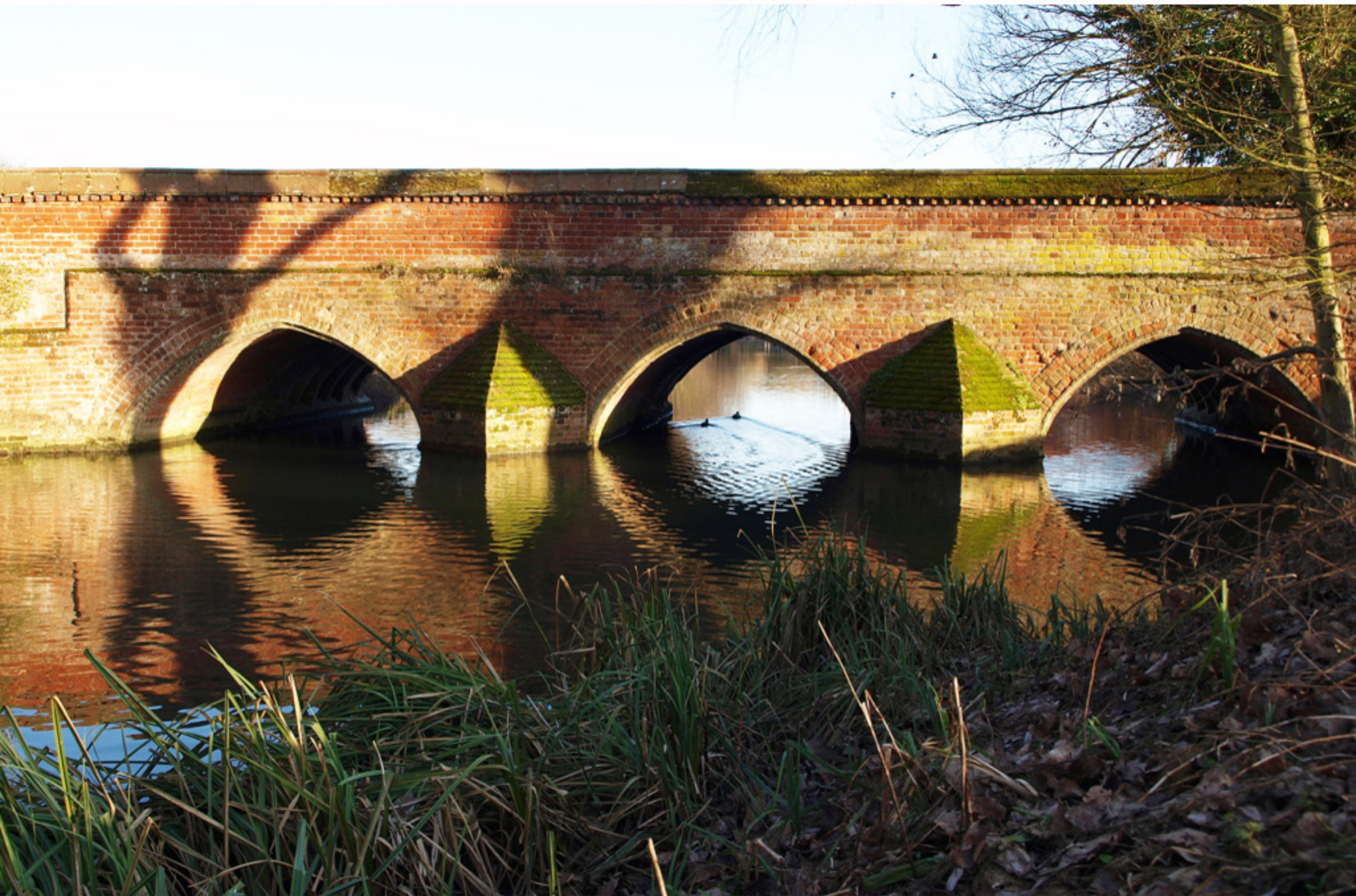
TOPPESFIELD BRIDGE, HADLEIGH, SUFFOLK
